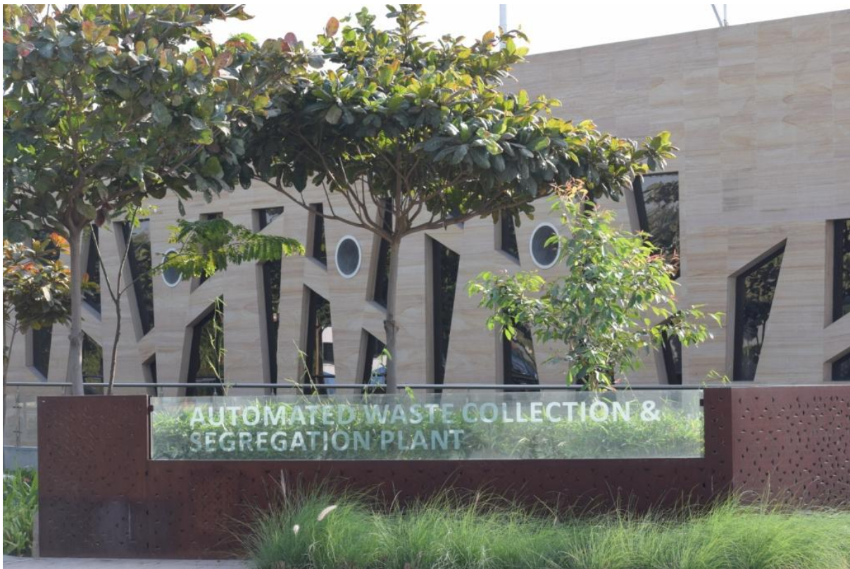
Automated waste collection segregation plant
